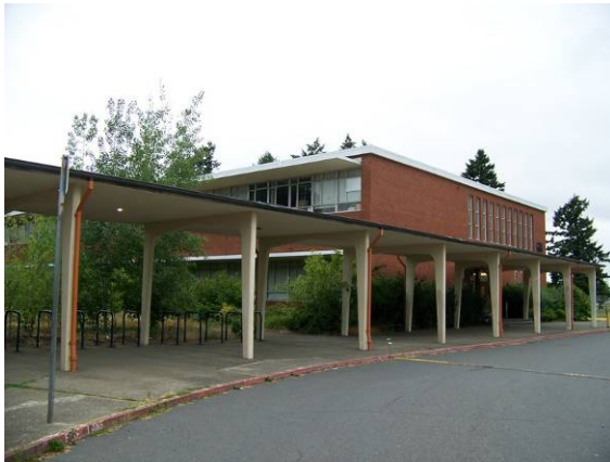
Main building (218A), east (side) elevation of the northeast wing and breezeway, looking northwest.
