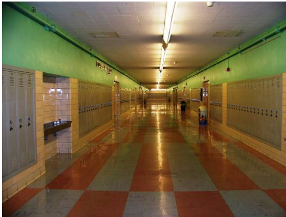
Main building (218A), southeast corridor, looking west.
