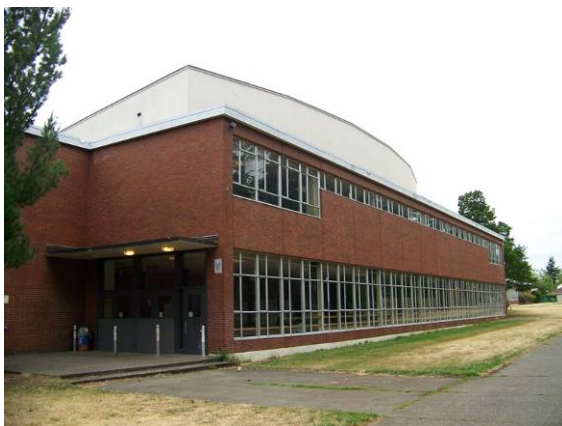
Main building (218A), north (front) elevation of the auditorium wing, looking southwest.
