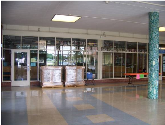
Main building (218A), lobby at the administrative offices, looking south.
