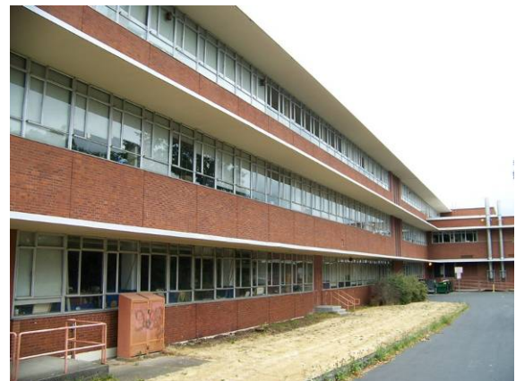
Main building (218A), south (rear) elevation of the south west wing, looking northeast.
