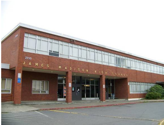
Main building (218A), north (front) elevation of southeast wing, looking southwest.
