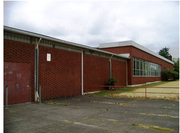
Main building (218A), north (front) elevation at the courtyard and cafeteria, looking southwest.
